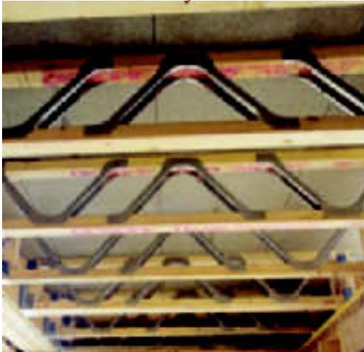
All types of pipework can run easily through Posi-Joist™ beams.
